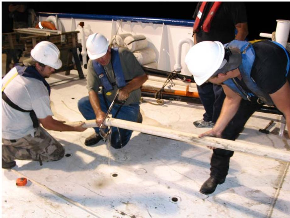
**Figure 5. CMRET technical team recovers a gravity core onboard the *R/V Pelican*.**
